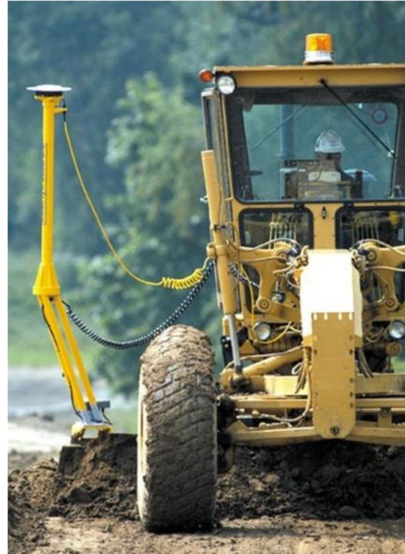
Figure 8: Motor grader with machine control.
