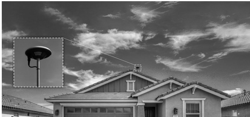
Image 2: Typical GEODNET Antennae Installation
