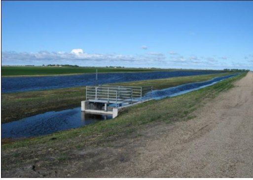
Structure C North Ottawa Impoundment
