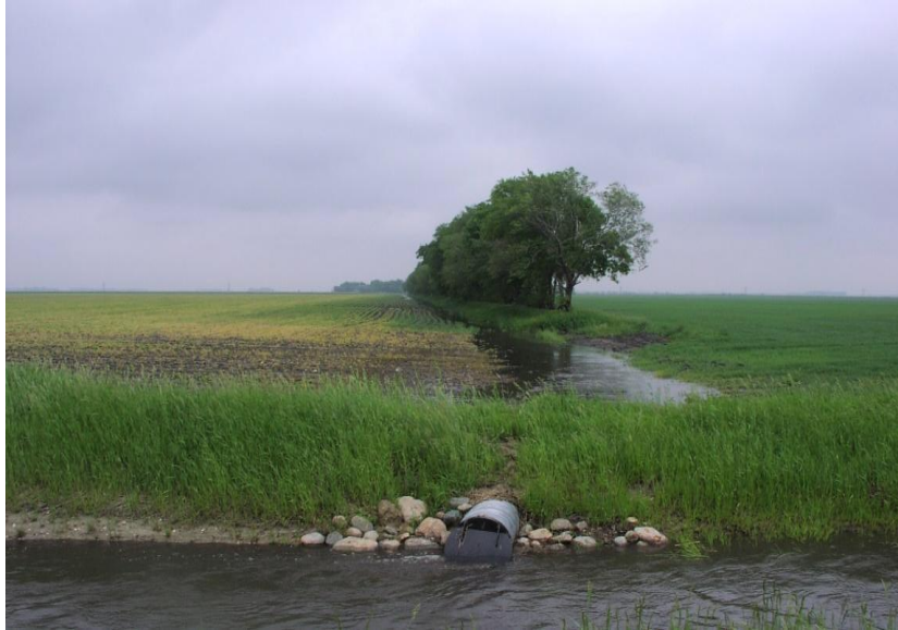
Wilkin County, Minnesota side water inlet
