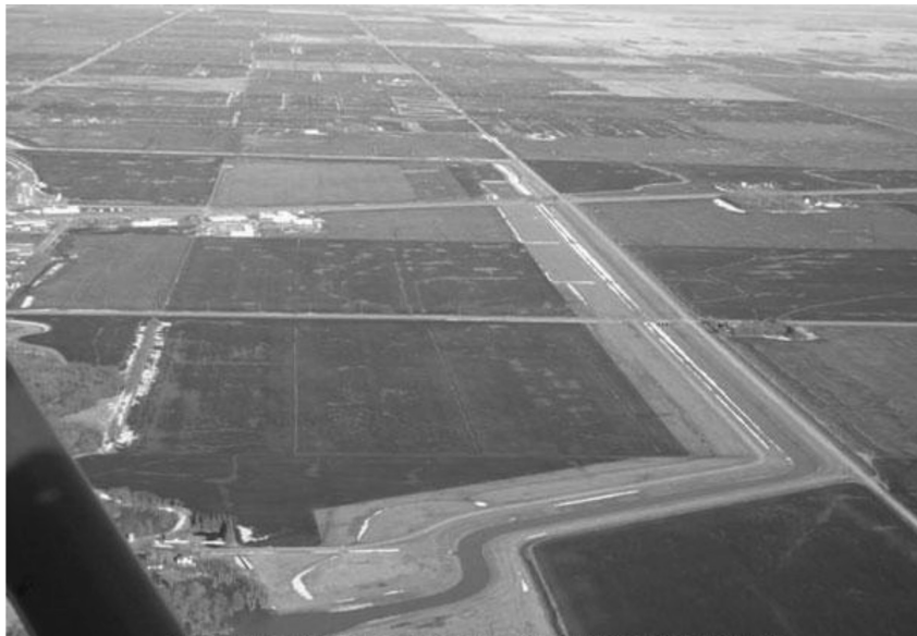
P.L. 83-566 Diversion Channel.
