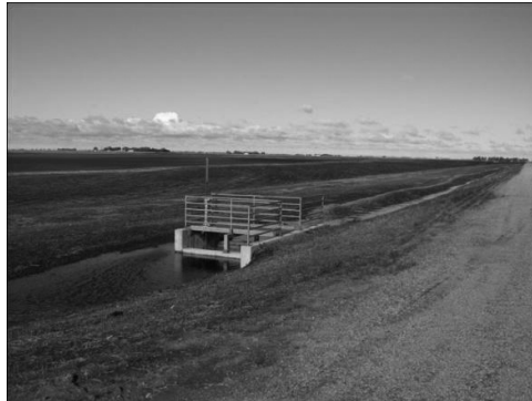
Structure C North Ottawa Impoundment.
