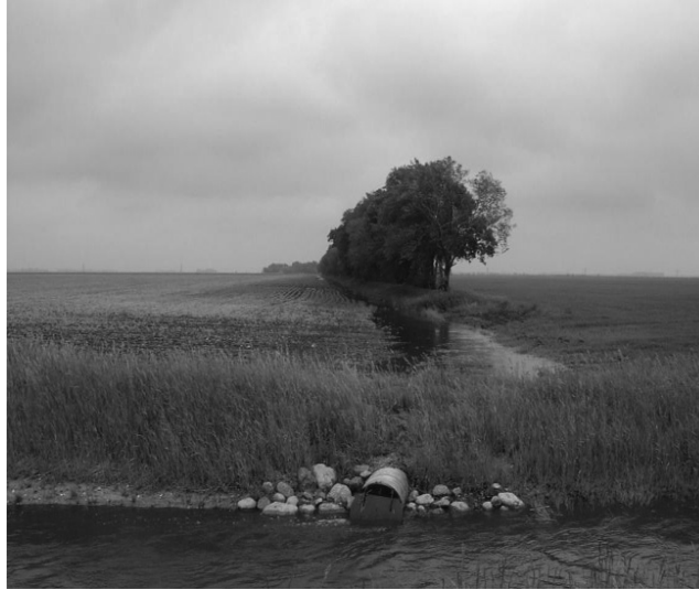
Wilkin County, Minnesota side water inlet.
